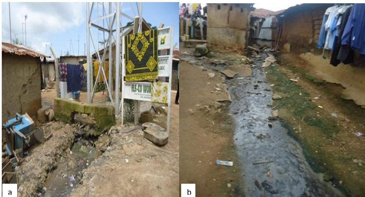
Plate 2(a&b): Discharge of leachate from unlined pit-latrines to the land surface
