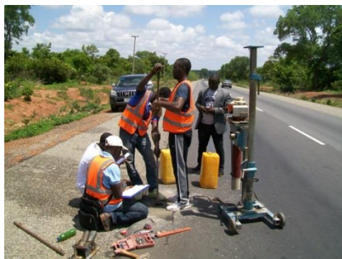
Fig. 4. Dynamic Cone Penetration test.
