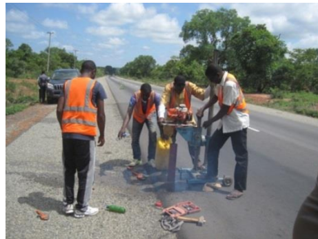
Fig. 2. Coring through the pavement structure..
