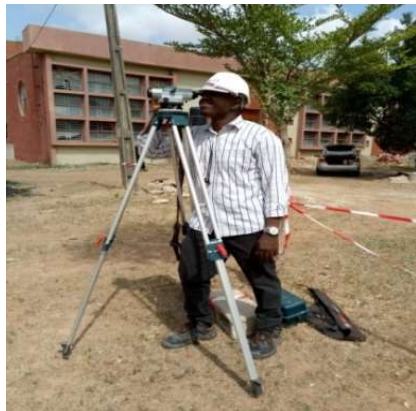
Fig. 6: Theodolite for leveling of subgrade
