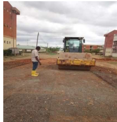
Fig. 8: Field compaction in progress
