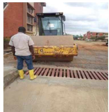
Fig. 9: Boundary with the existing pavement
