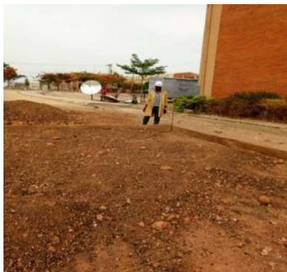
Fig. 7: Sections demarcated with planks
