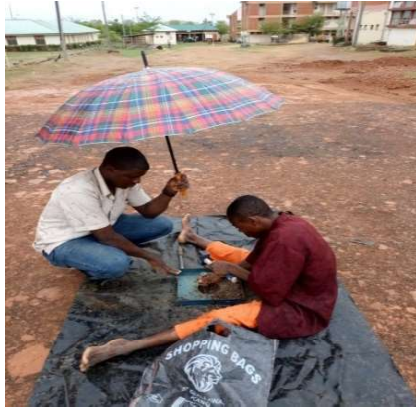
Fig. 10: In-situ density test on the road surface
