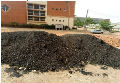
Fig. 2: Pile of milled RAP
