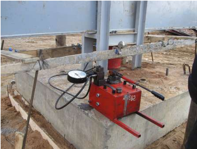
Fig. 1 Hydraulic Jack (200T capacity) for loading
