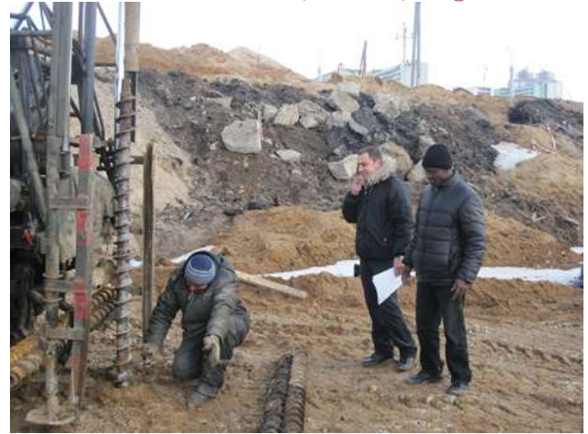
Fig. 4 Boring during the Field Test
