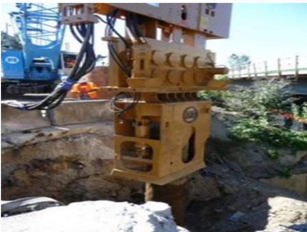
Fig. 3 Vibratory Pile Hammer during Field Test
