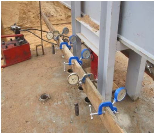
Figure-5: Dial gauges for Settlement Reading
