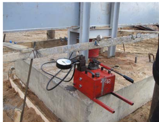
Figure-4: Loading device of 200T capacity
