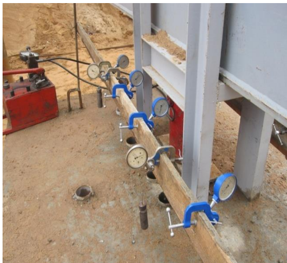
Figure 5: Dial gauges for Settlement Reading
