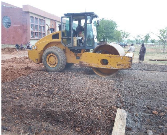
Plate IV: Field compaction of laterite-RAP mix
