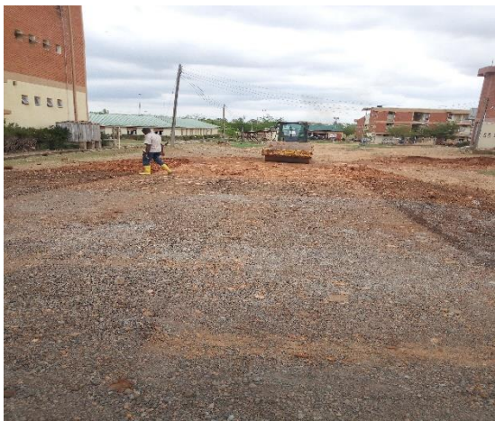
Plate III: Field compaction of laterite-RAP mix
