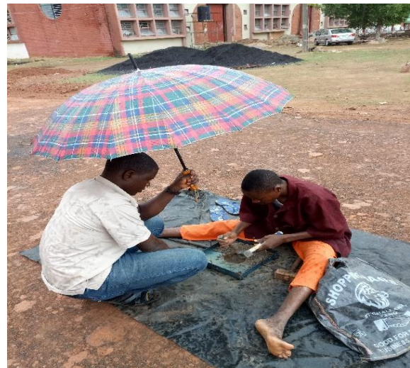
Plate VI: In-situ density test of RAP
