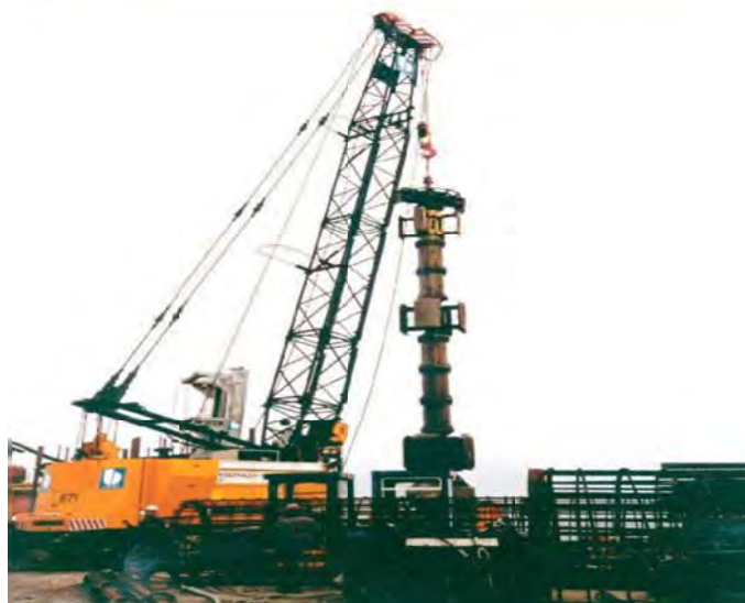
Figure 3: A multi- purpose pile installation Rig
