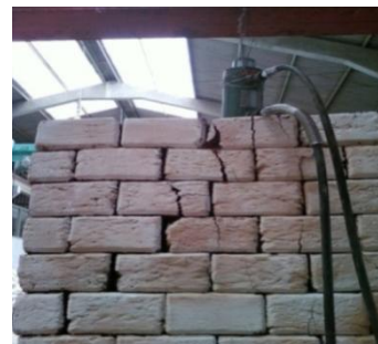
5(b): Failure of un-stabilized wall
