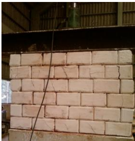
Fig 6(a): Un-stabilized Murang'a soil wall
